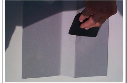
Step #6: Once the putty is dry to touch use a brush to dab resin over the repair to give a textured look to the repair area.
