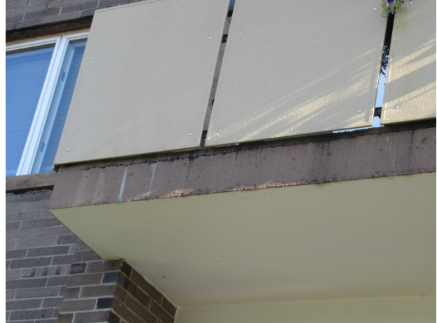
Efflorescence
