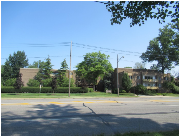
Front (south) elevation overview
