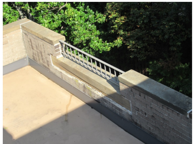
Repairs at balcony stone sill
