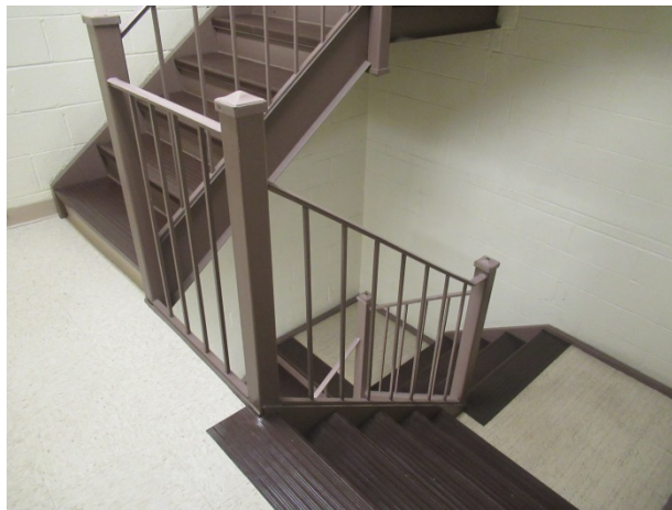
Vinyl at staircase
