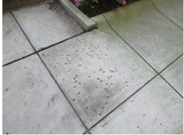
Concrete spall
