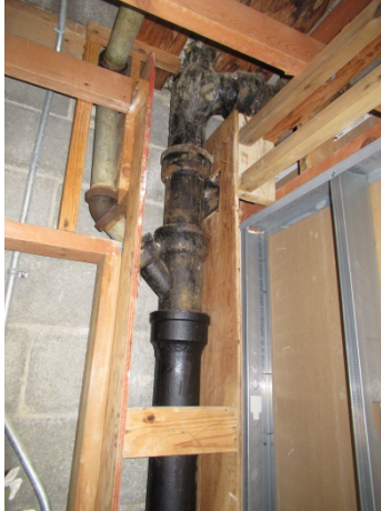
Location of pipe repair at part room 'build-out'
