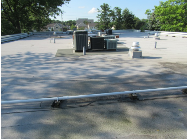
Modified bitumen overview
