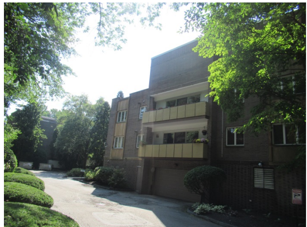
Rear (north) elevation overview
