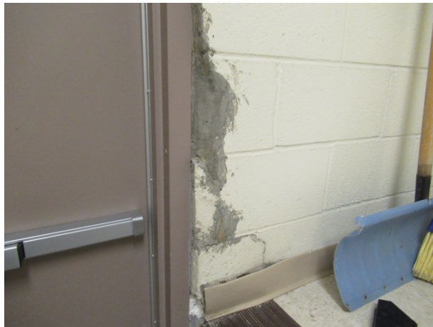
Stairwell wall repairs
