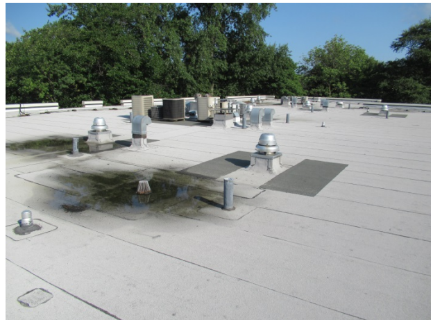
Roof overview, note ponding water and build-up at drain
