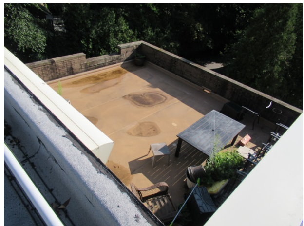
Membrane at balcony
