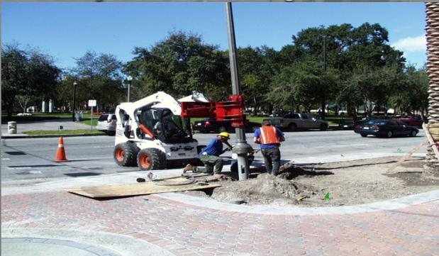
"These machines allow co-op line workers to set new poles or replace downed poles in areas of limited access. They are well-suited for storm restoration be it blizzard, tornado or hurricane, to help line crews work safer and more efficiently."
