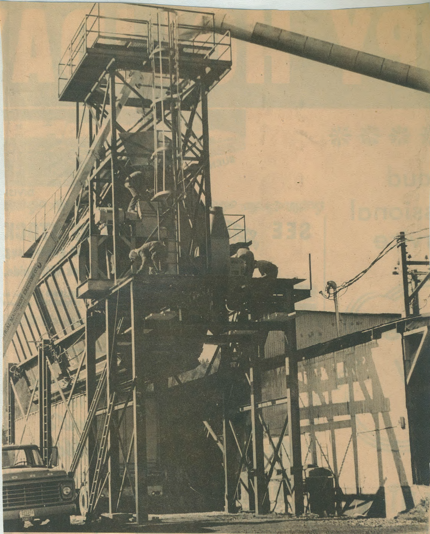
CONTRACT WORKMEN are installing fractionizer, which will reduce shavings to sawdust and thus create additional market for Vanport Mfg. products.
