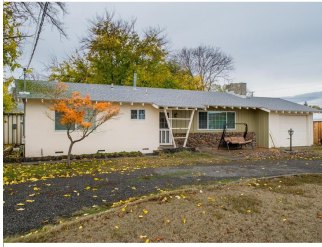
1310 East Street Home Orland, CA
