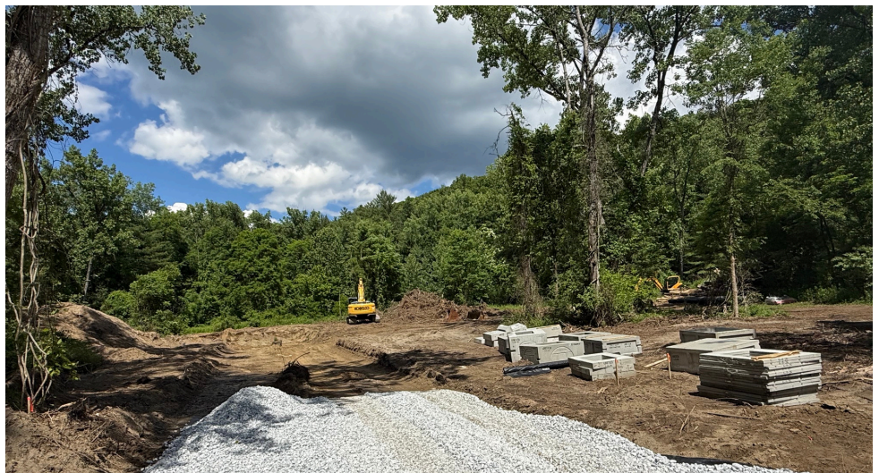
Site work has begun at the River Road property.
