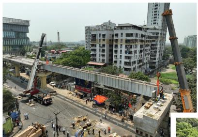
OKA- Khidirpur section of JOKA-Esplanade Metro runs along the median of extremely busy Diamond Harbour Road. There was a big challenge to launch the 50m span on this road at the T-junction called Burdwan crossing. To accomplish this feat, two road-mounted cranes - one weighing 250 tonnes and another weighing 150 tonnes - were utilized, with an additional 300-tonne crane on standby.
