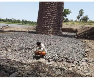
uring a period of heavy rainfall, Bridge number 134 faced significant erosion and damage to its pier foundation. The constant downpour caused severe scouring around the pier, eventually exposing its foundation. To address this issue and safeguard the stability of the pier, protective measures were taken. A Gavion
