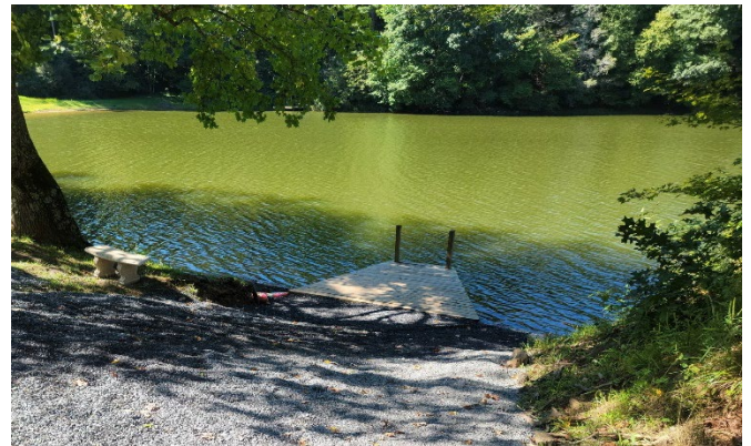
Finished dock access ramp.
