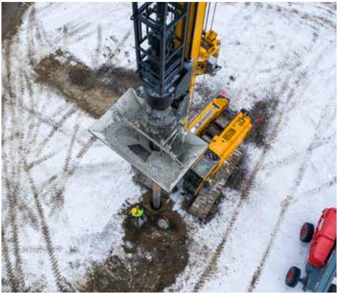
Kiewit Foundations installed 1,022 non-vibratory stone columns at the new Kiewit Headquarters in Omaha, Nebraska. Each is 24 inches in diameter with a depth ranging from 20 to 30 feet. Kiewit is the only contractor that has installed non-vibratory stone columns in North America.
