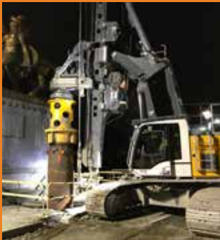
DRILLED SHAFTS
