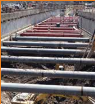
STRUCTURAL SLURRY WALLS/CEMENT BENTONITE PANELS
