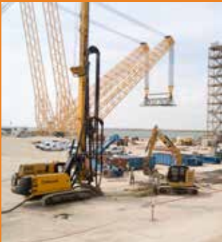
ACIP/DISPLACEMENT PILES
