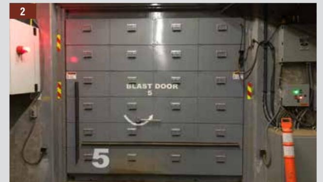
1. The project team engineered new equipment that could move on an incline, in a horizontal direction, within the existing ore pass. 2. Six blast doors were installed to keep air pressure, air flow and blast effects away from an existing laboratory on the 4850 level. 3. Many pieces of equipment were disassembled to fit in the hoist system and later reassembled underground.
