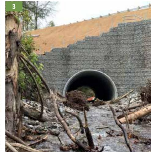
1. The old concrete culvert was replaced with this 26-foot diameter multi-plate round steel culvert. 2. To keep traffic moving, crews built a 180-foot-long temporary bridge to span the creek. 3. This photo shows the nearly-completed project. Trees and shrubs were planted in the stream banks, and will eventually create a more natural look.
