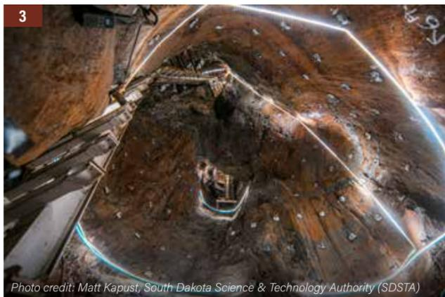
1. The new conveyor system was installed over U.S. 85. 2. When complete, the conveyor system will have the capacity to move 400 tons of rock per hour. 3. The reclaimed and rehabilitated ore pass from the historic mine works will now be used to transport excavated rock to make way for massive underground caverns.
