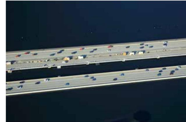
*When the LRT project opens in 2023, the 105-foot-wide top deck of the bridge will allow for a pedestrian path, four lanes of vehicle traffic and two directions of light rail track, eastbound and westbound. The westbound track will be complete by summer 2020.*
