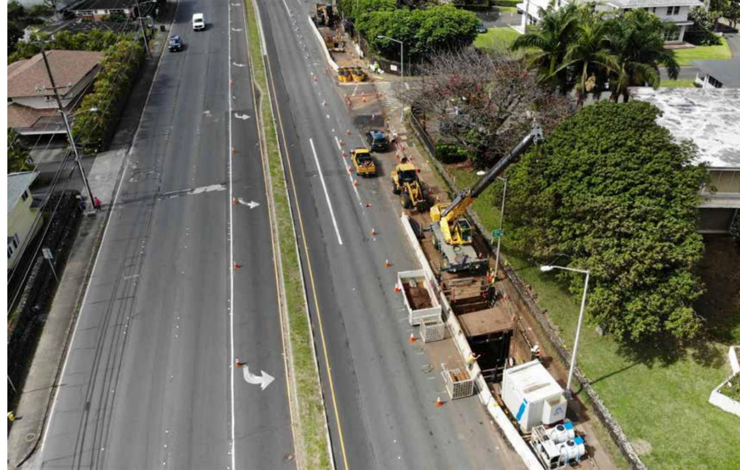
*The Dowsett Highlands Sewers Project required installation of 17,500 linear feet of new gravity sewer lines, using guided bore and open excavation methods.*
