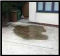
**Pooling Water** - Pooling water on the concrete isn't good news. It means there is likely sinking or shifting beneath that is causing the concrete to hold precipitation and impede drainage. Since concrete is a porous material, it's best not to have standing water on it for long periods, so raising the slab surface to facilitate drainage might help.
