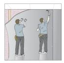
**POSITION MLV AND BEGIN FASTENING**With a helper, position the first cut piece of MLV. Begin fastening starting from the top of the wall working your way down.
