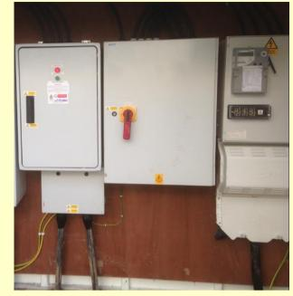
There are spare ways/capacity available in the existing 6-way 250A 3-phase TP&N board - on the existing array – **the 3-phase volt drop at this DB (PV DB1) 6-volts**.
