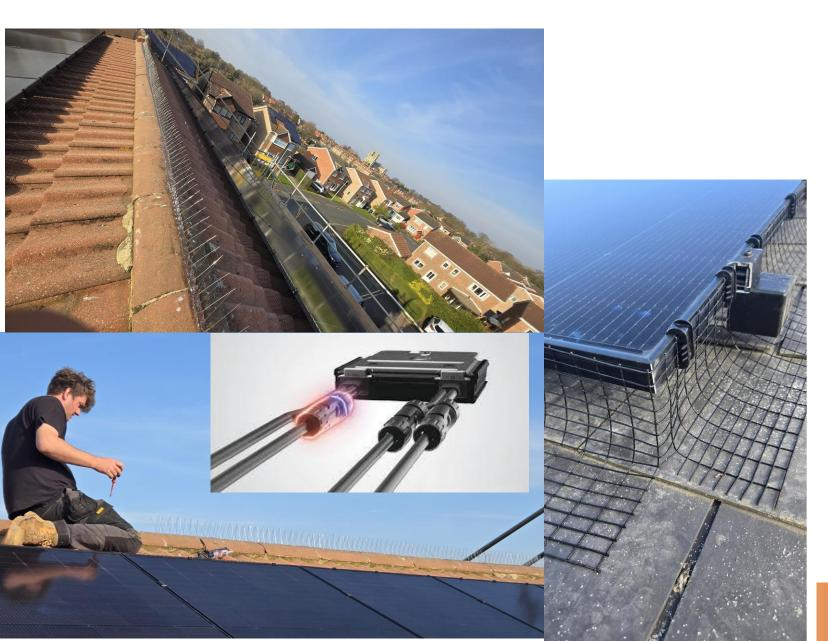
Bird guard which retains air flow, is metal coated and provides a safe zone under arrays to protect the protective measure of double/reinforced insulation. Along with wider bird/rodent deterrents.
