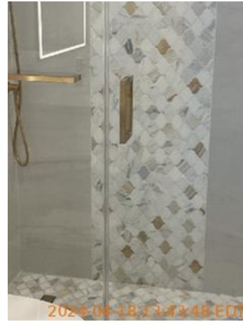
2024-04-18 13:43:48 EDT Shower Door/Rail/Curtain □ 2024-04-18 13:43:48 □ 25.82946749613477 , - 80.1207648761902 □ Image
