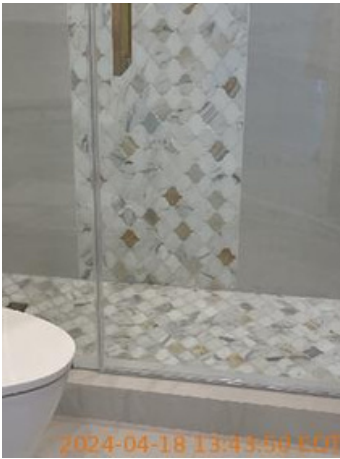
2024-04-18 13:43:50 EDT Shower Door/Rail/Curtain □ 2024-04-18 13:43:50 □ 25.82946749613477 , - 80.1207648761902 □ Image
