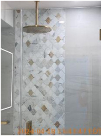
2024-04-18 13:43:47 EDT Shower Door/Rail/Curtain □ 2024-04-18 13:43:47 □ 25.82946749613477 , - 80.1207648761902 □ Image
