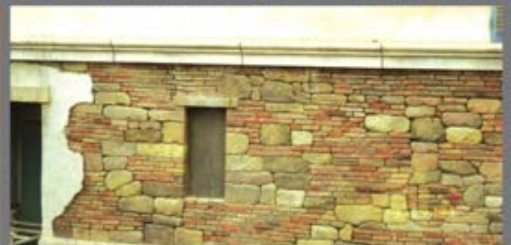
Application of 32,000m 2 Carved Stone Face Plaster. Installation of 4200m 2 Stamped Colour Concrete.
