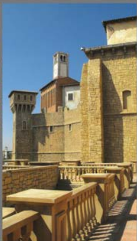
Installation of 800m 2 Themed Artificial Rockwork. Decorative GRC like Coping and Arches.
