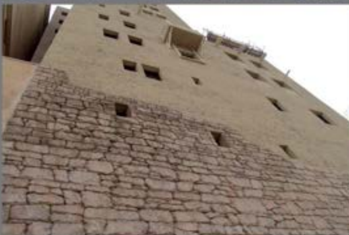
Installation of 1000m 2 Themed Artificial Rockwork. Application of 600m 2 Stone Face Plaster
