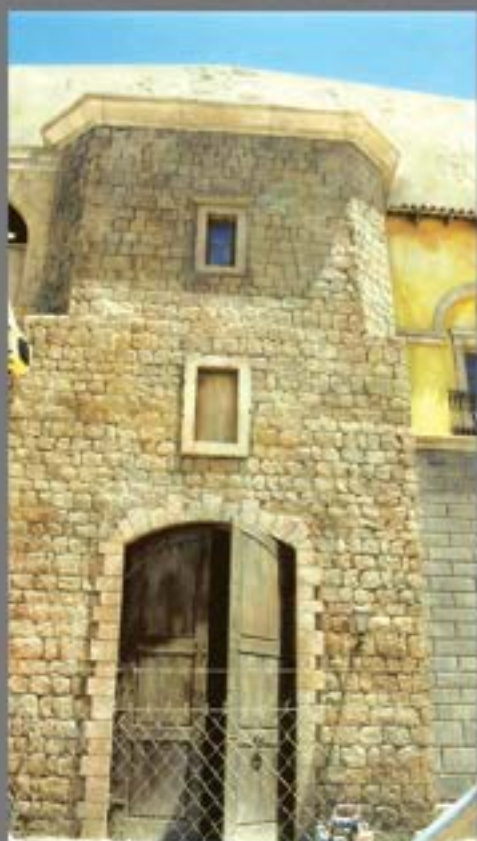
Installation of 800m 2 Themed Artificial Rockwork. Decorative GRC like Coping and Arches.
