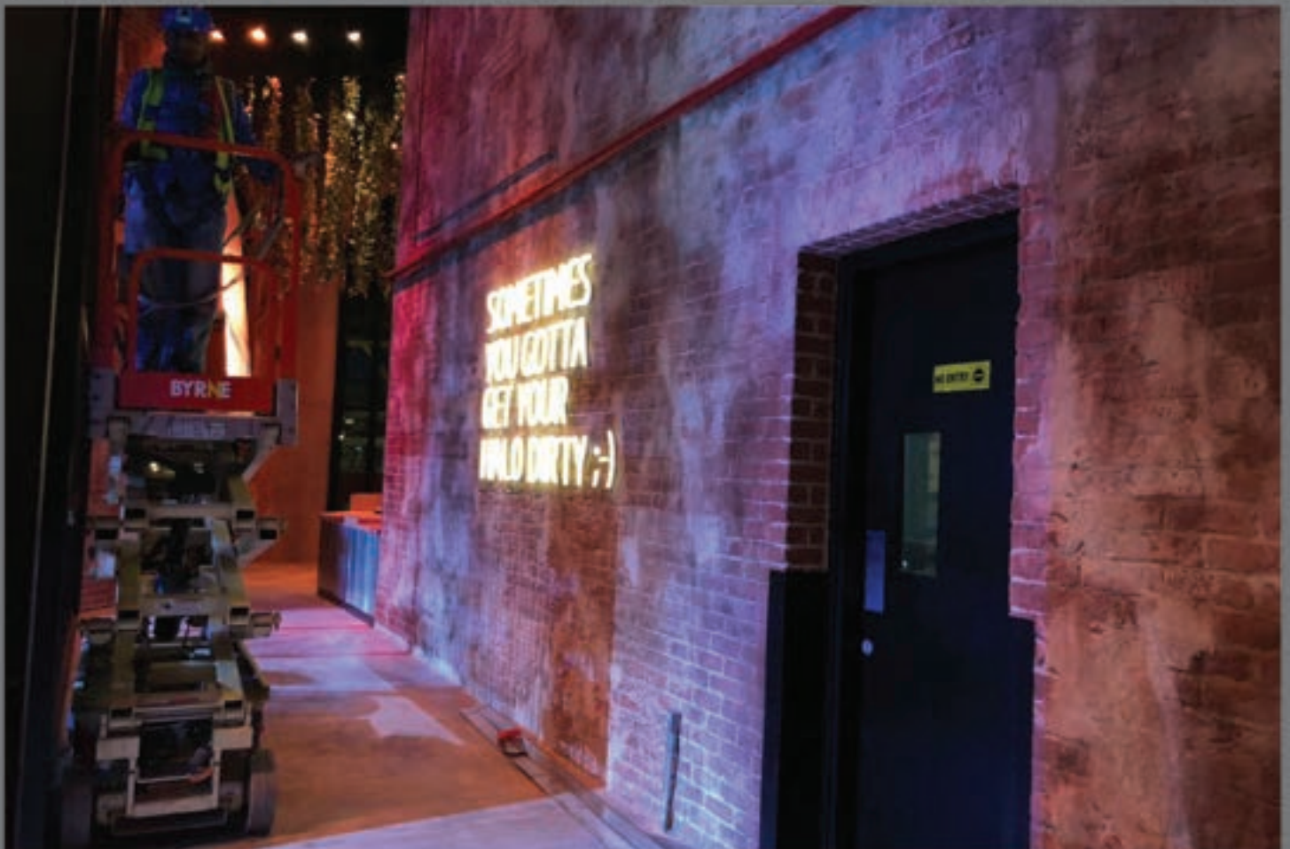
Installation of Bricks Style Themed Plaster
