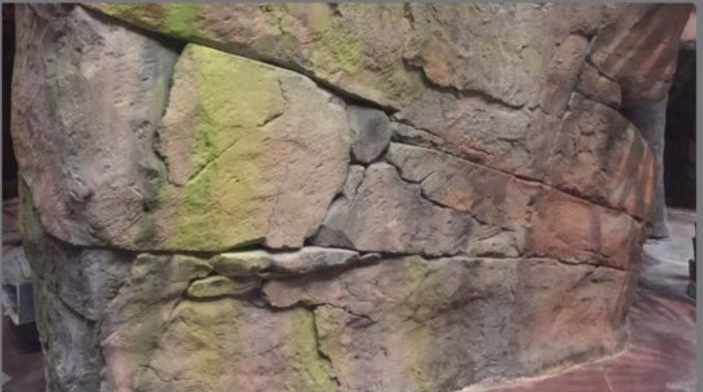
Installation of Positive Rock work
