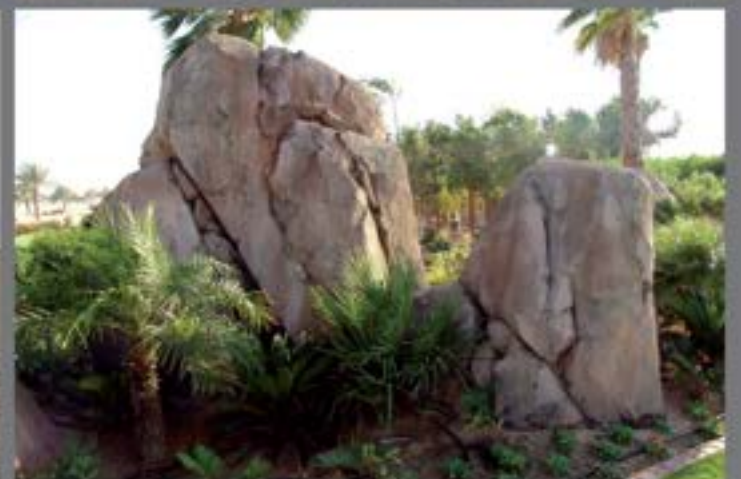
Installation of 1000m 2 Themed Artificial Rockwork. Application of 600m 2 Stone Face Plaster
