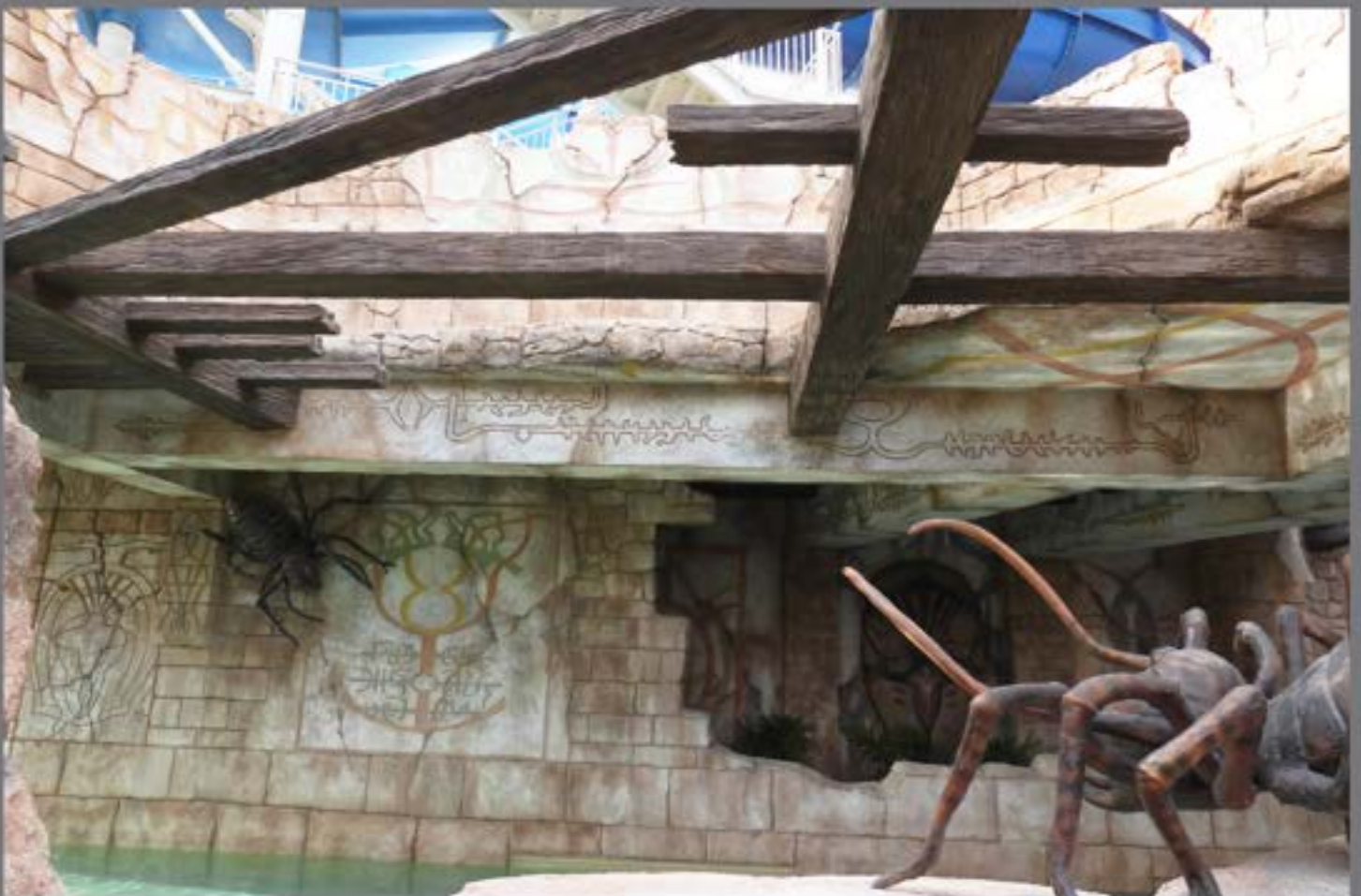
Structural Steel Pergola with GRP Timber Theme Cladding and Stone Face Plaster
