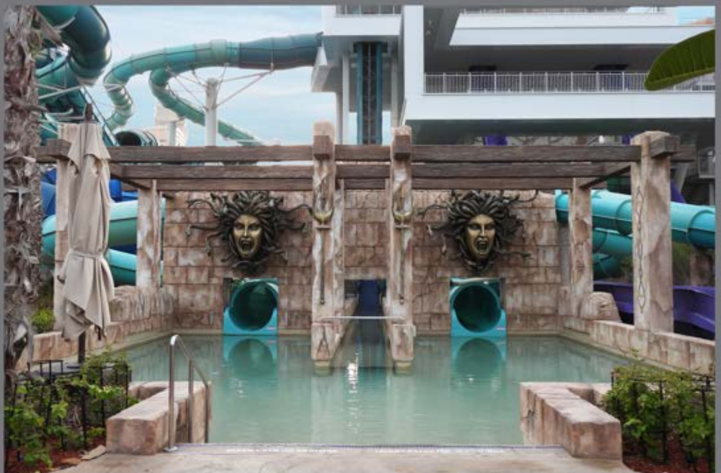
GRP Medusa Sculpture, Structural Steel Pergola with GRP Timber Theme Cladding and Stone Face Plaster
