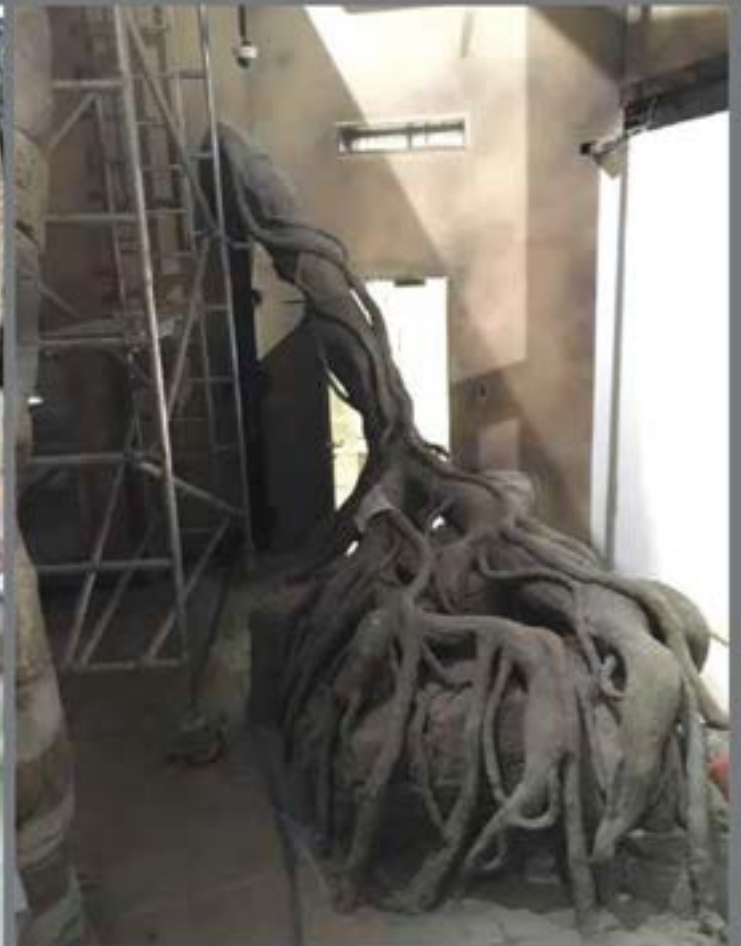
Artificial Carve plaster Tree and Rock work
