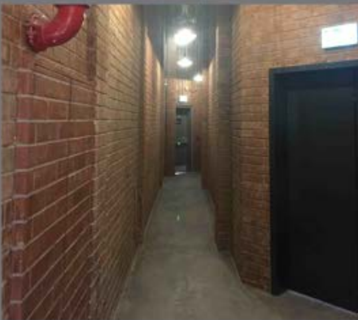
Application of Stoneface plaster and Stamp Concrete
