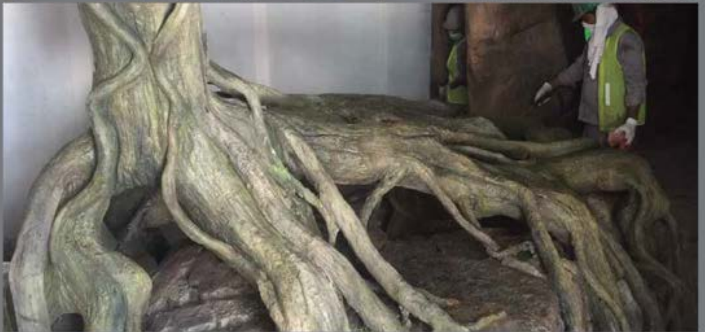
Artificial Carve plaster Tree and Rock work
