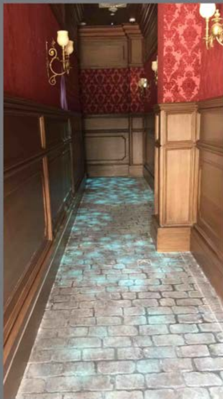
Application of Stoneface plaster and Stamp Concrete
