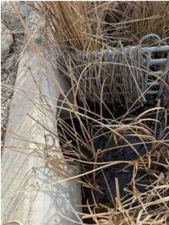
30" dia Pipe Culvert near Cetus Drive
