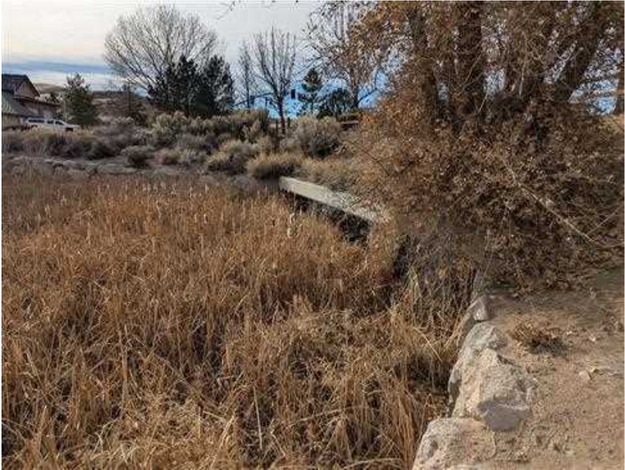
Vista Culverts, 3 cell 12'x4'
