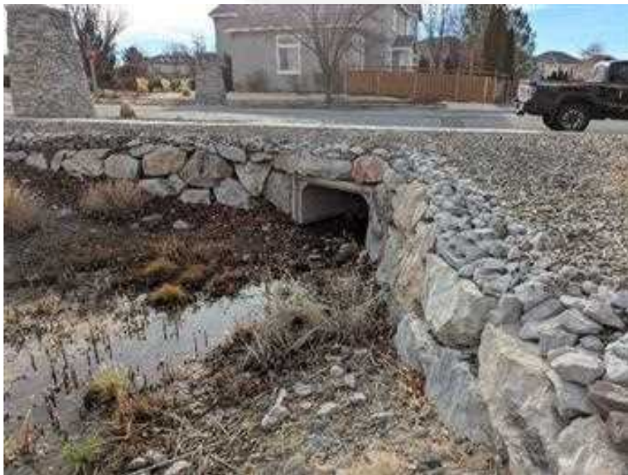
RCB culvert near Little Easy Street and Decoy Dr.
