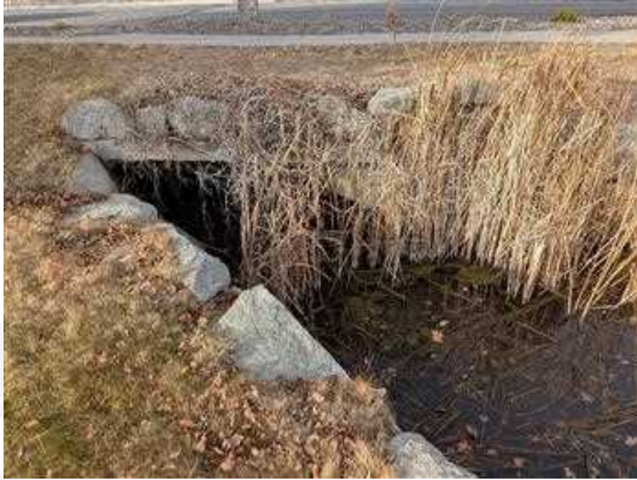
8'x4' RCB Culvert under General Thatcher Dr.
