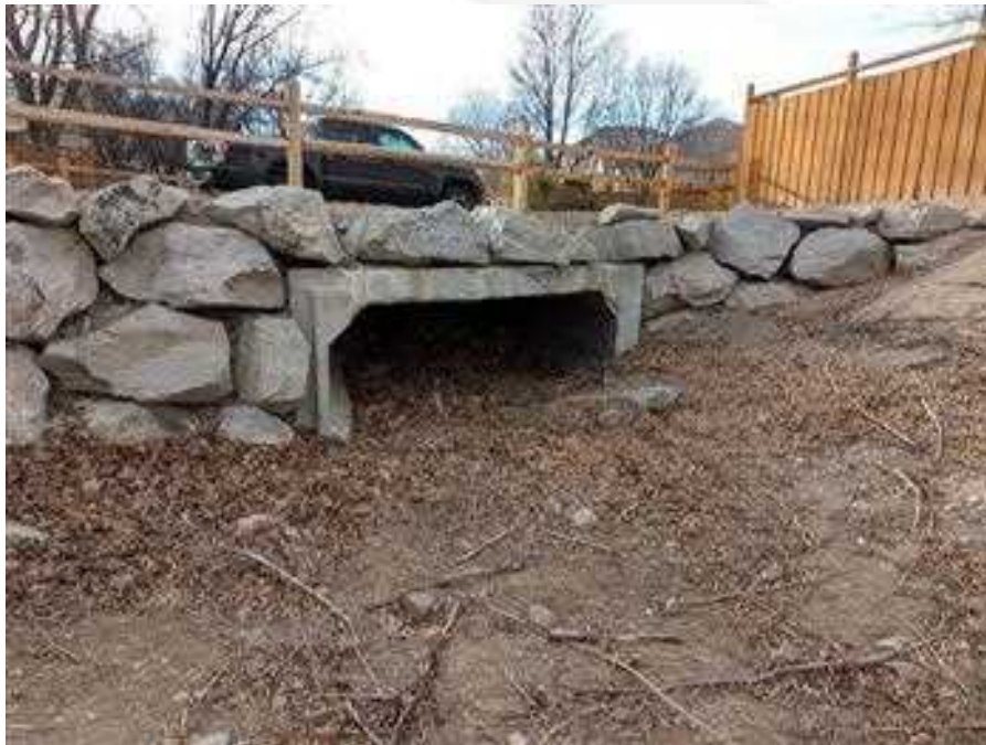
12'x4' Box Culvert under Wingfield Springs Rd near Poco Bueno Dr
