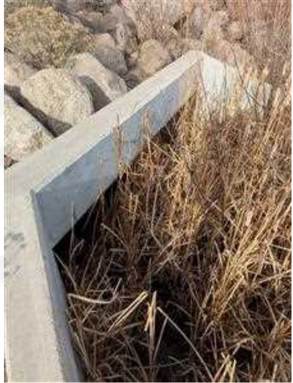
12'x4' RCB culvert near Cetus Drive
