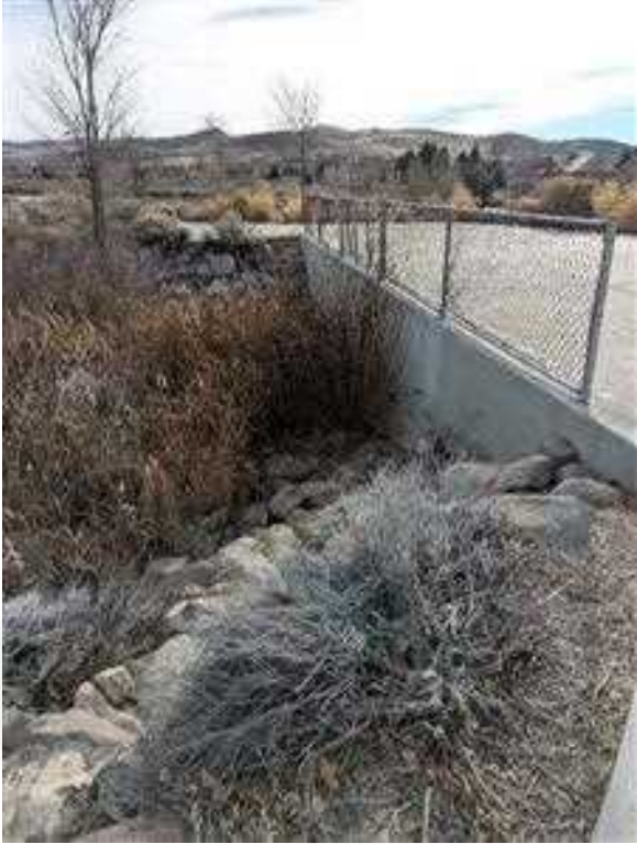
30" dia Pipe Culvert near Cetus Drive
