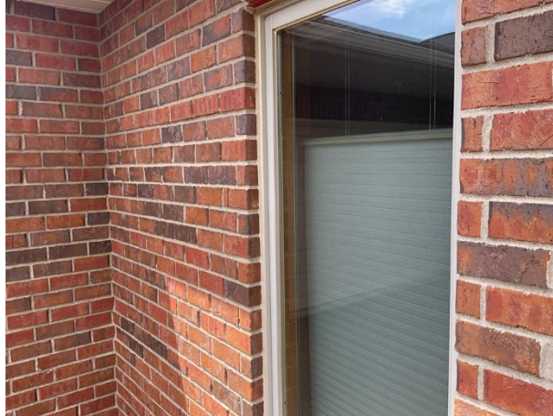
Sealant in good condition
