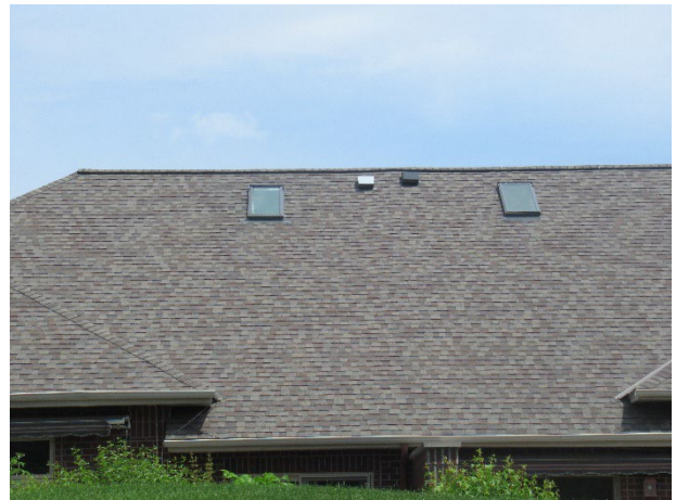
Asphalt shingle roof overview
