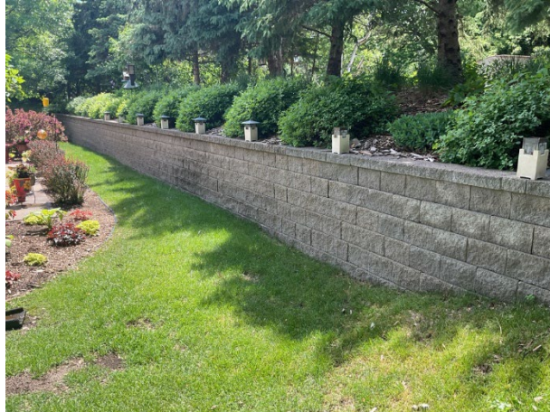
Masonry retaining wall at Units 129 and 135
