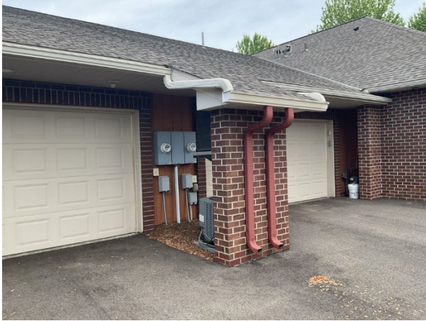
Aluminum gutters and downspouts
