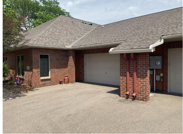
Aluminum gutters and downspouts
