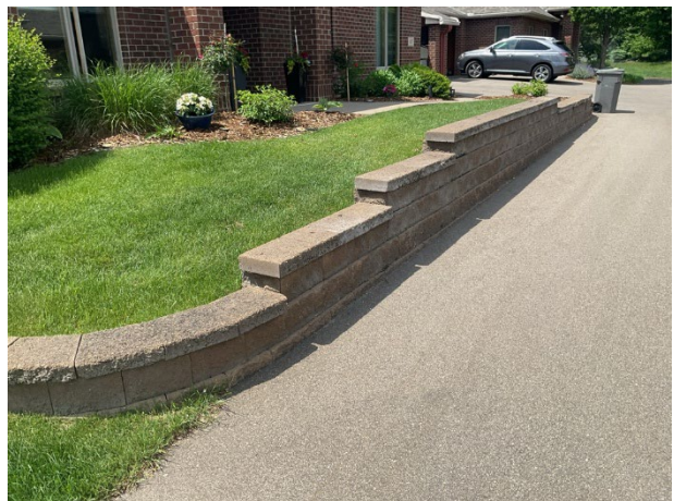
Masonry retaining wall
