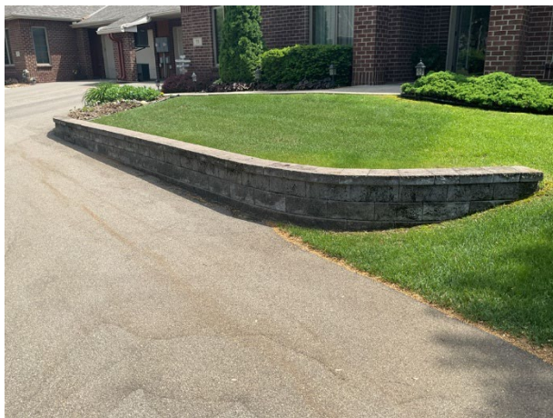
Masonry retaining wall
