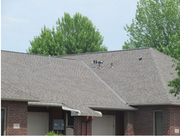
Asphalt shingle roof overview
