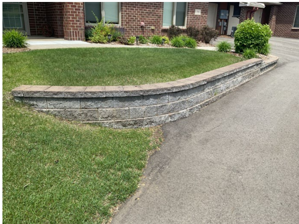
Masonry retaining wall
