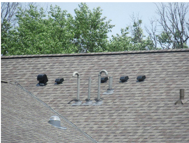
Penetrations and square hood box vents
