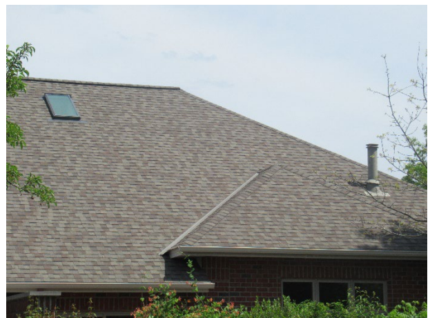
Asphalt shingle roof overview
