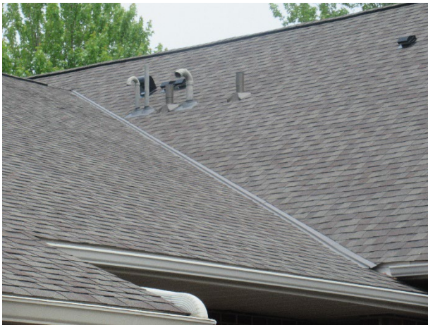
Open valley with metal W flashing
