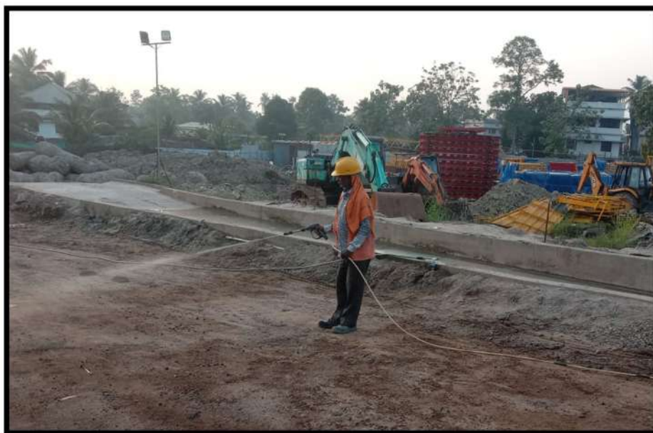
Photograph of the Water Sprinkling
