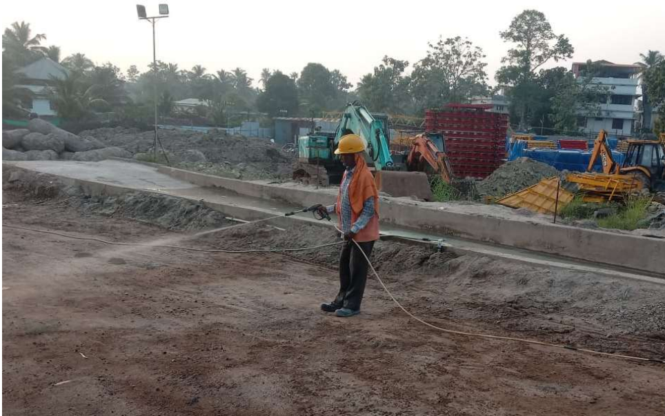
Photograph of the Water Sprinkling
