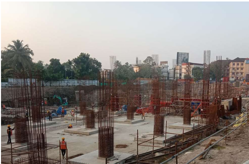
Photograph of the Project site
