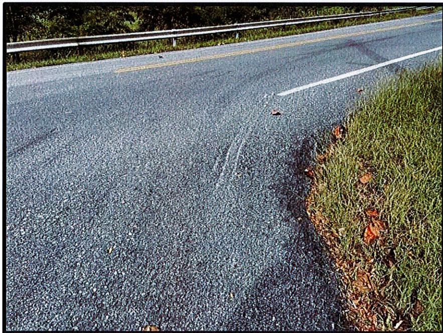
Figure 5: Intersection Wheel Paths
