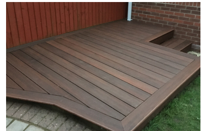
Bullnose Boards used to define the edge of the deck
