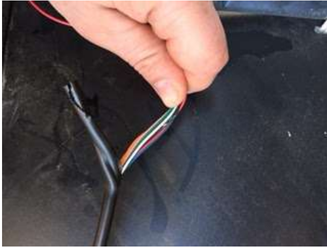
Figure 6 - Cable shielding stripped back 6"
