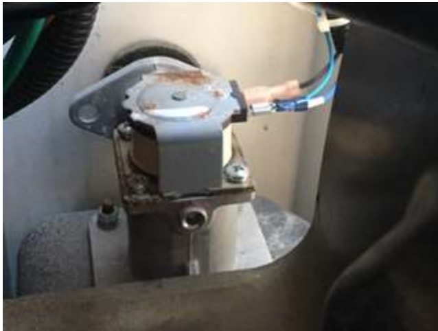
Figure 16 - Generator running connected to fuel solenoid
