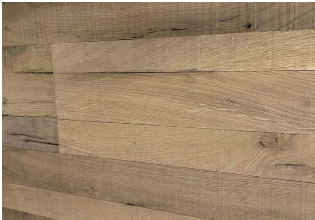
WOOD FLOORING UPGRADE
