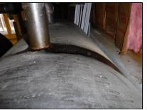
**Observation:** The oil tank did show signs of leaking. I did not note any patching of the tank. The leaking seemed to becoming from the top fill pipe. I would place this tank near the middle of its expected life cycle.
