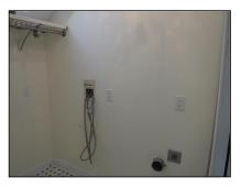
(1) **Observation:** I did note that the dryer is vented to the outside. The washing machine was not operated at the time of the inspection. Therefore, I was unable to test the washing machine drain. The standpipe was the correct size.
