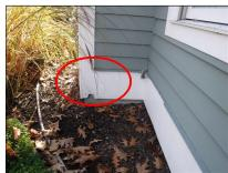
**Observation:** Portions of the wood trim throughout the house exhibit signs of deterioration, especially along the skirt board and drip cap located below the first course of siding.
