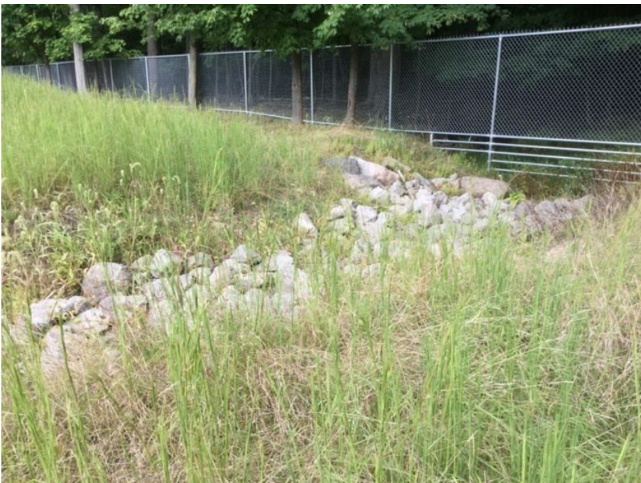
View of emergency spillway located in the northeastern portion of the basin.
