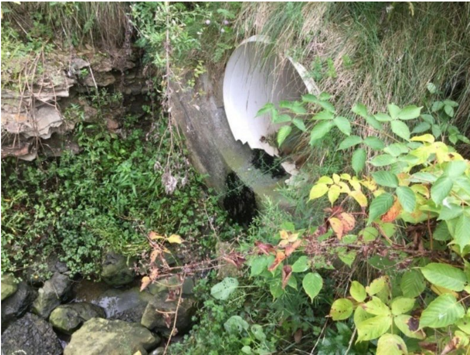
Up close view of damaged inflow pipe in the southeast.
