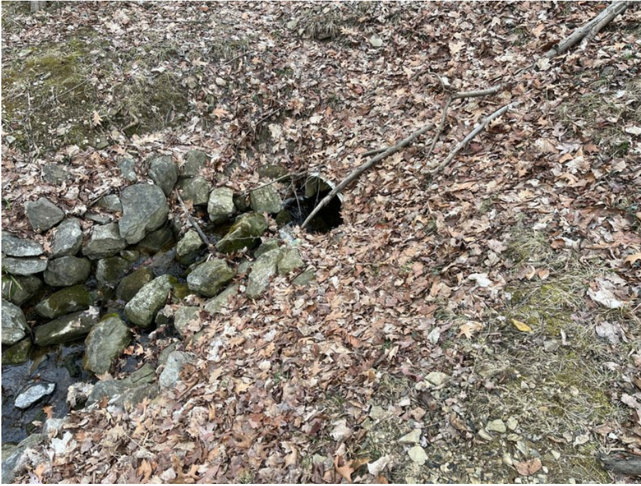
View of outlet outfall. Remove any debris.
