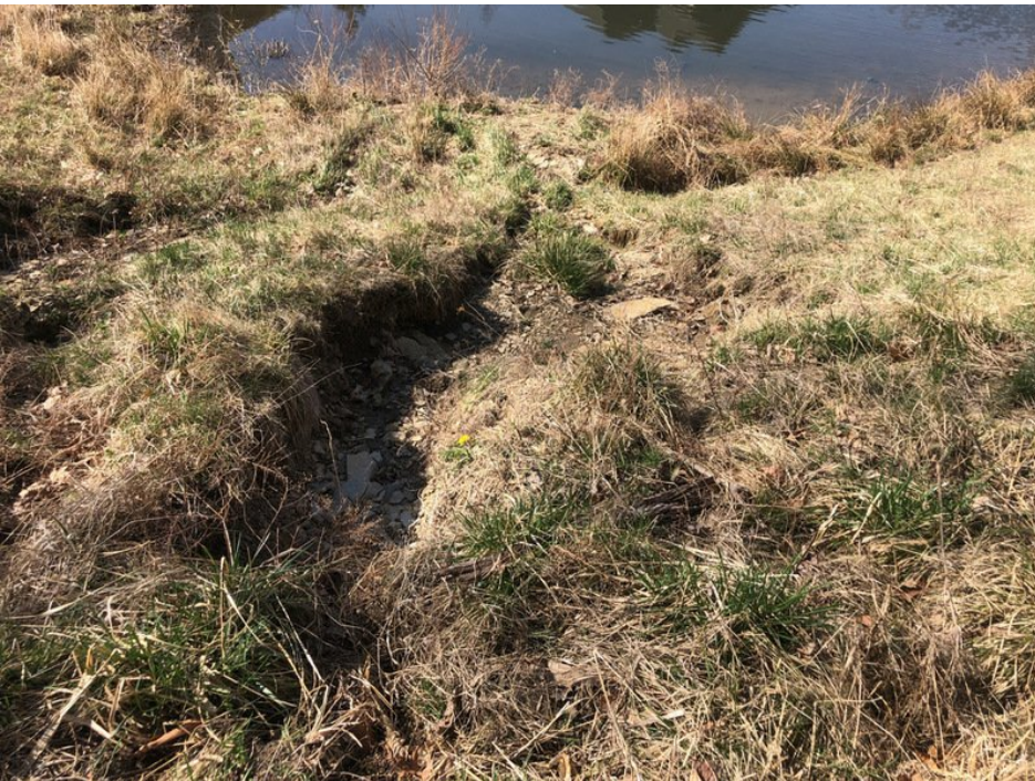
View of erosion rill. Check around the basin for other erosion rills or bare areas that need to be stabilized.
