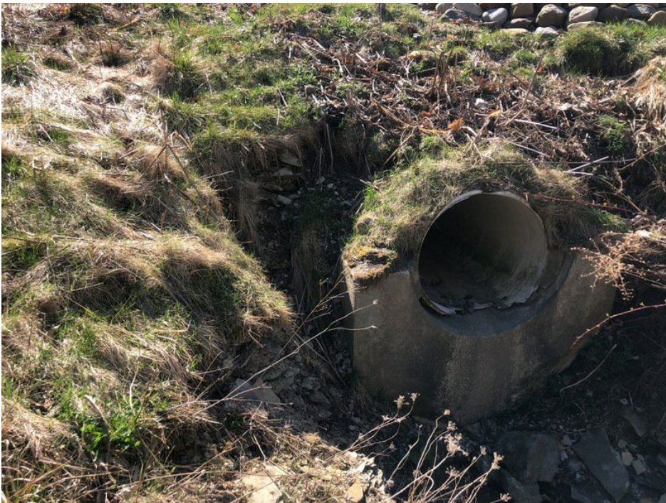
View of the headwall erosion.
