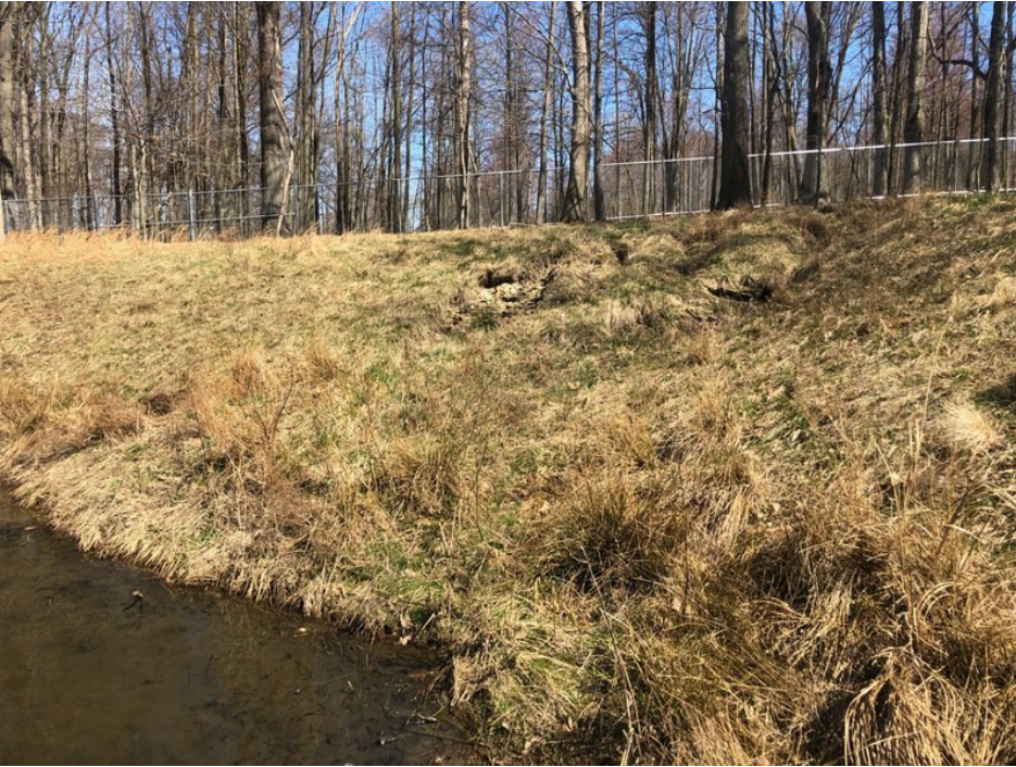
View of erosion rills in the basin berm. This needs to have soil added and be re-seeded.
