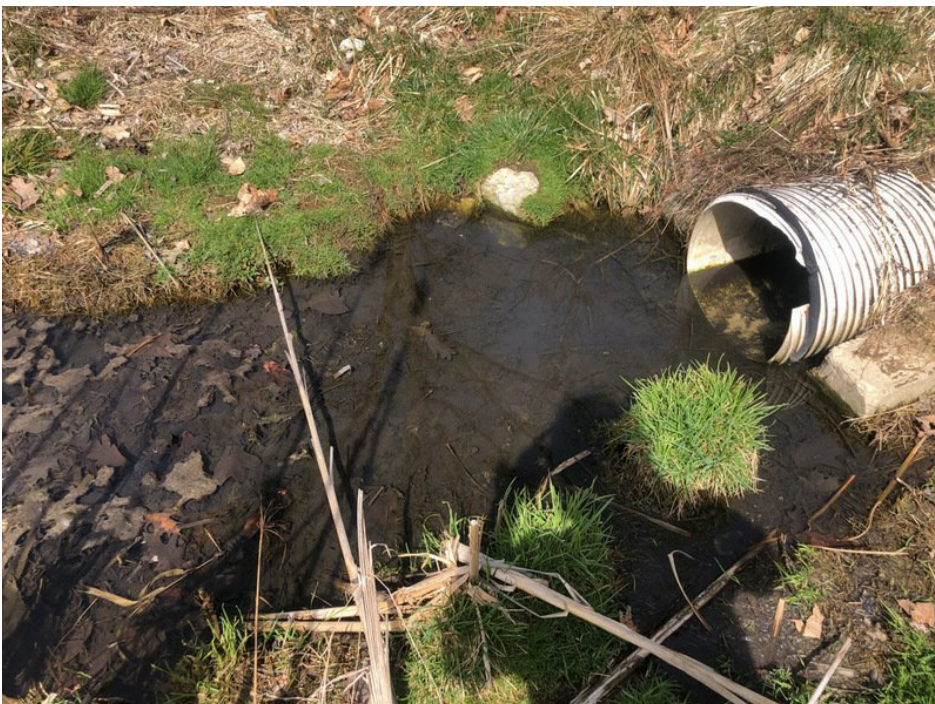
View of sediment accumulation in the basin. This needs to be dredged soon.
