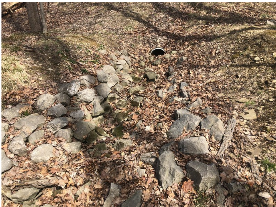
View of outlet structure covered with leaves. There was also minor erosion/slumping around the outlet structure.
