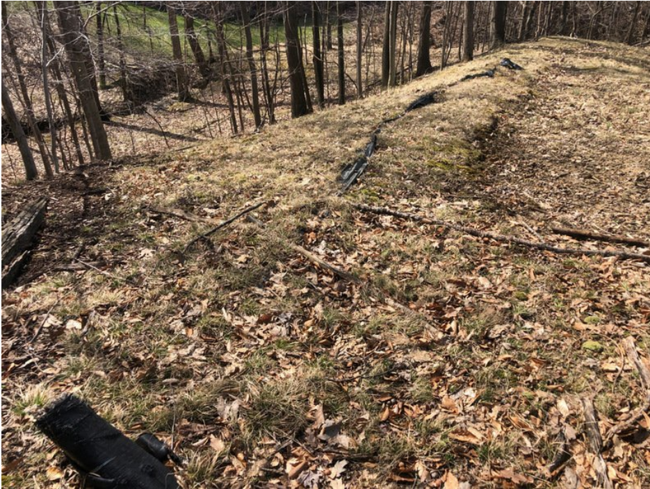
View of silt fence. This needs to be removed.
