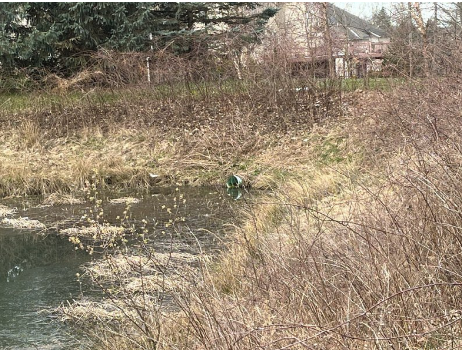
View of outlet structure.
