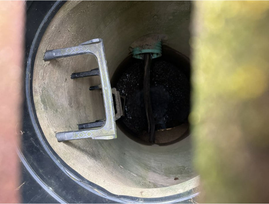
View inside outlet. Clean out debris.
