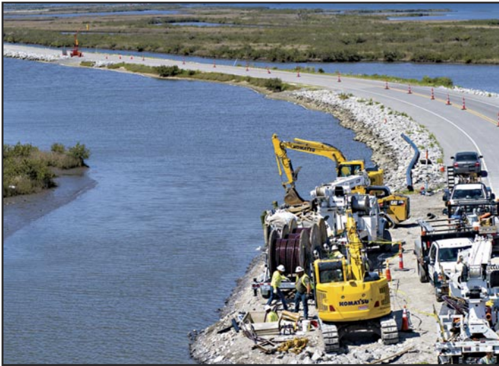
Workers undergrounding a portion of the distribution system in Grand Isle.
