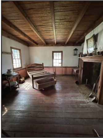
The Hypolite-Bordelon Home is over 200 years old. It was built with hand-hewn timbers in traditional Creole style.
