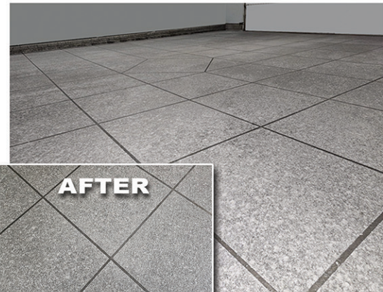
Below is the finished garage floor. And it is guaranteed not to delaminate, unlike other products that will delaminate
