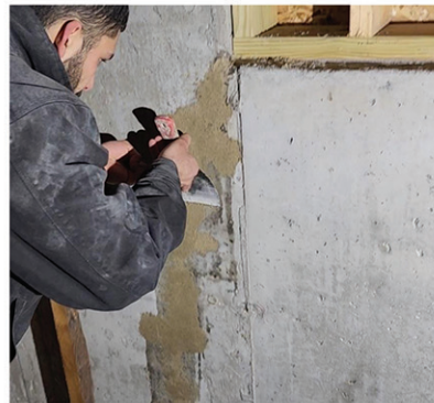
We patch with CONCRETE FUSION Concrete Repair Product
