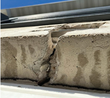
CONCRETE LINTEL Before Patching
