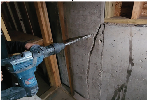
We drill holes for our Staple System
