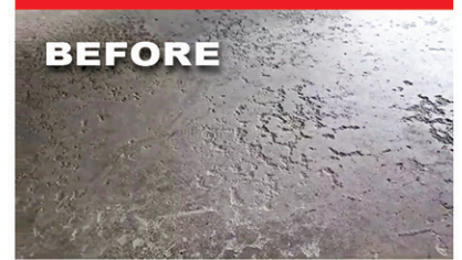
We can repair garages that have been ruined by the salt, where the cream of the concrete has been destroyed. (sample above)
