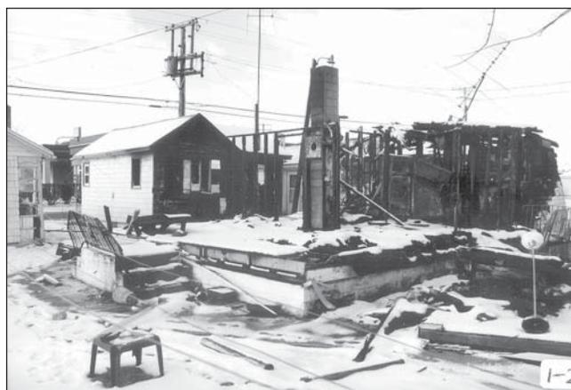
Figure 1 – Wood Frame Home Remains after Natural Gas Explosion
