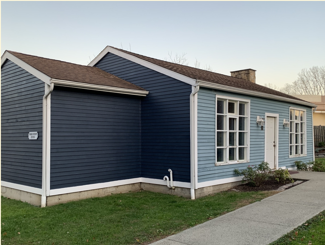
A little before and a little after as we repaint the Marian Anderson Studio.
