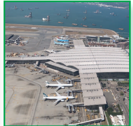
Hong Kong International Airport
