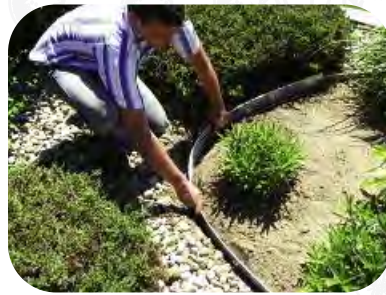
2. PLACE EDGING IN TRENCH
