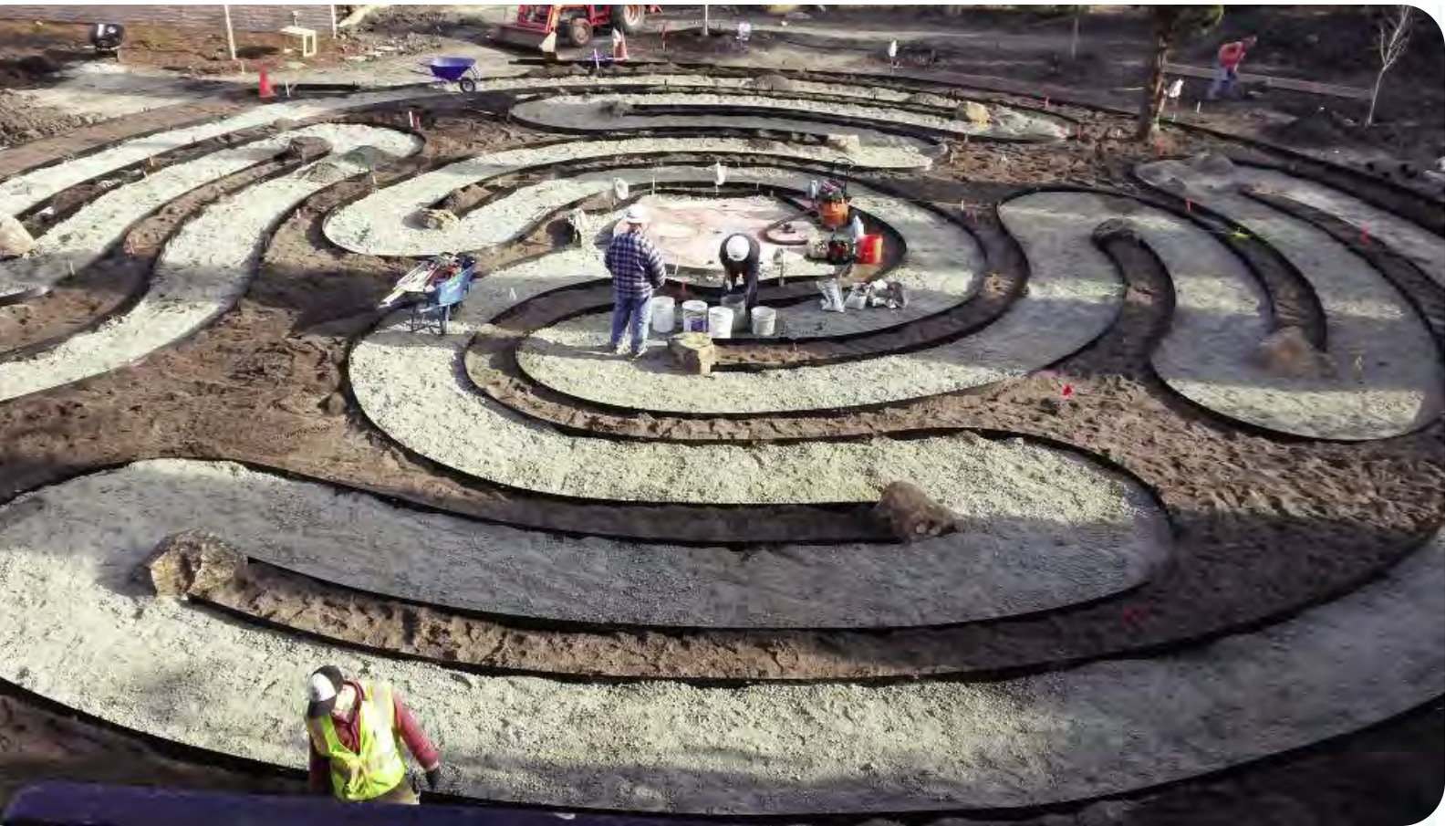
Work in progress, using Sure-loc Black Anodized Aluminum Edging. Note the fluid curves and defined spaces.
