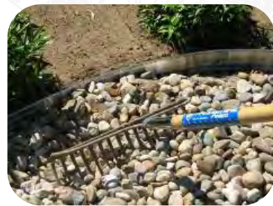
5. BACKFILL 1/2' BELOW EDGING
