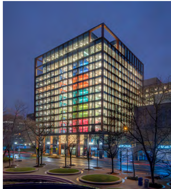
Confidential Commercial Building in Crystal City, VA LEED Platinum Certified © Sam Kittner
