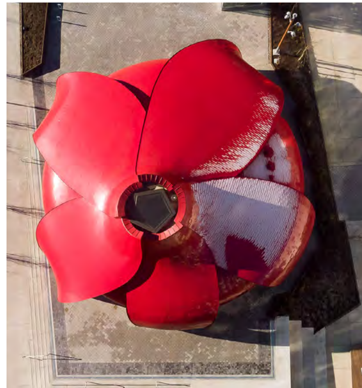
Great Northern Way Pavilion, photo courtesy of Keith Panel Systems
