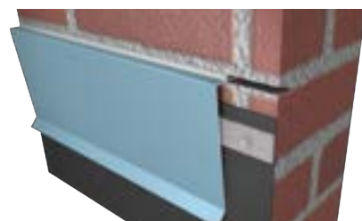
1-piece Counter Flashing
