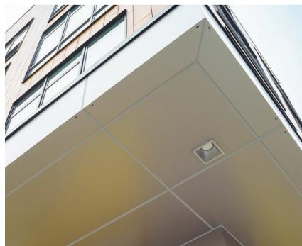
A backer rod and silicone caulk is used to fill the channels and seal them, making the ECONNECT-Z™ impervious to water. Various colors of caulking can be used to achieve the desired aesthetics of the facade. The use of silicone caulking makes ECONNECT-Z™ an ideal panel system for curved panel applications.
