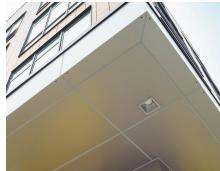
A backer rod and silicone caulk is used to fill the channels and seal them, making the ECONECT-Z™ impervious to water. Various colors of caulking can be used to achieve the desired aesthetics of the facade. The use of silicone caulking makes ECONECT-Z™ an ideal panel system for curved panel applications.
