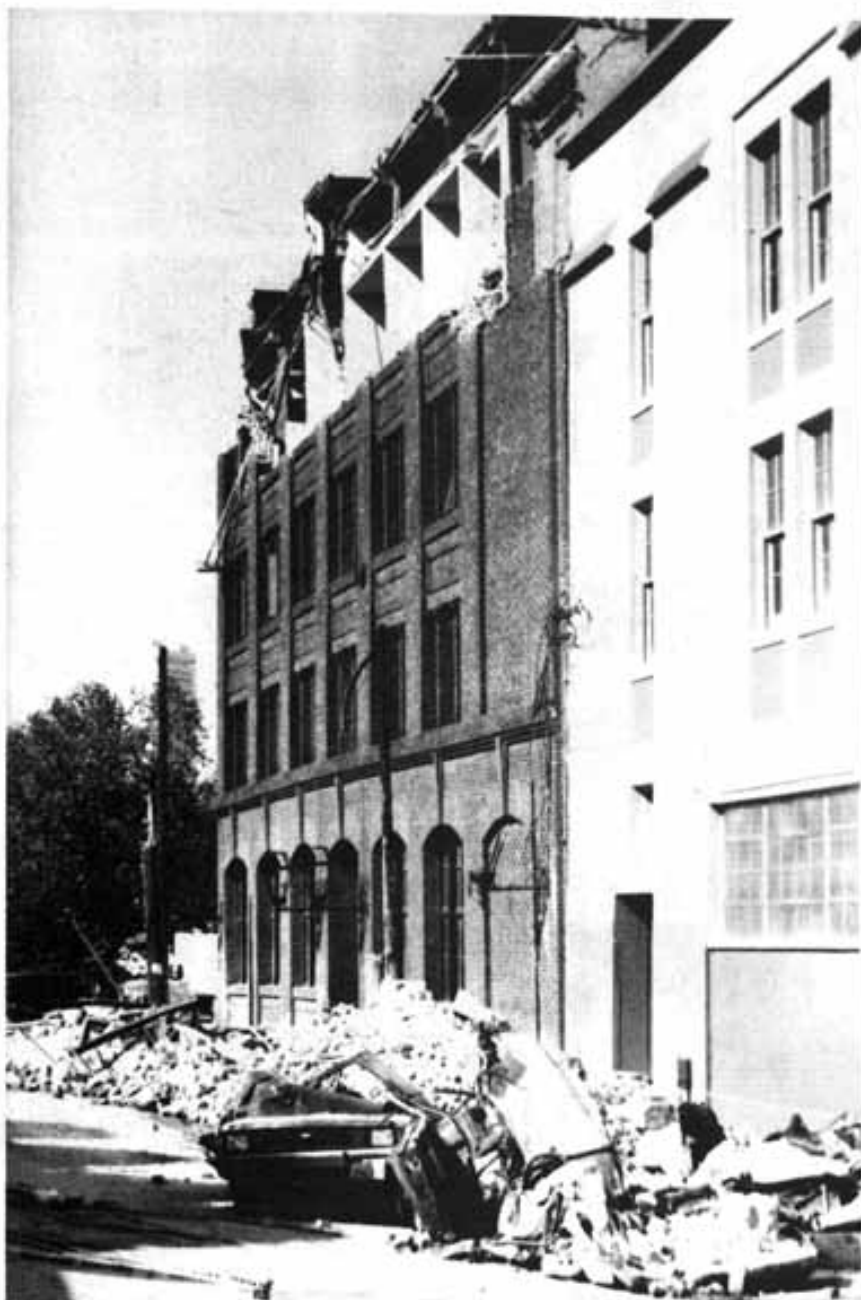
SHAKY TIMES Fatal building collapse on Bluxome Street
