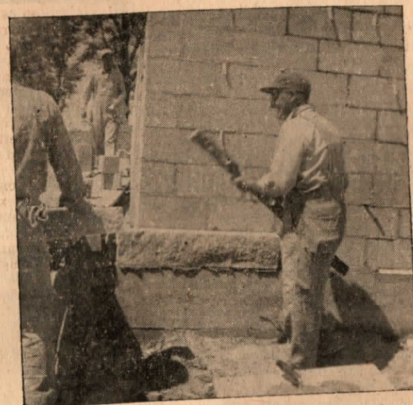
Mr. Clark, the stone contractor, lays the first of many Bedford stone in the structure. All photos through the courtesy of Hugh H. Goudie.
