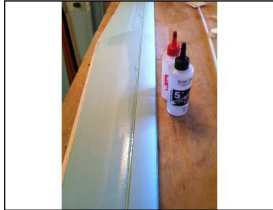
Figure 7 Properly installed fiberglass rod!
