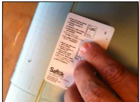
Figure 5squeeze the epoxy into groove and around rod
