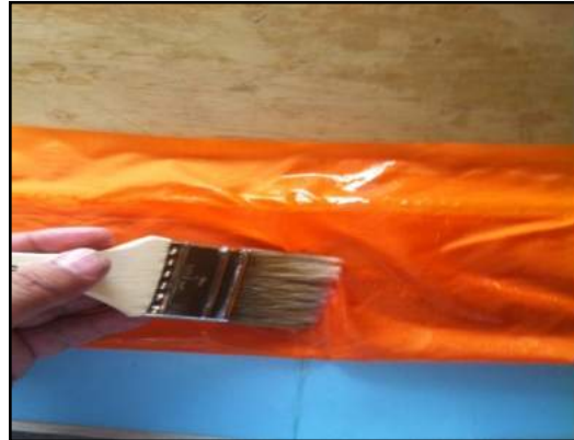
Figure 13 Coat-out fabric
