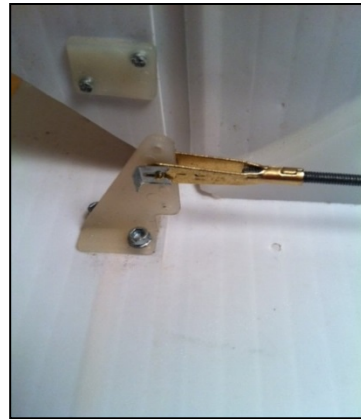
Figure 57 elevator control horn close up
