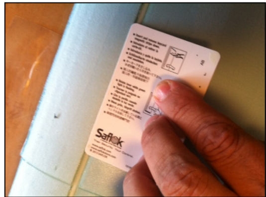
Figure 5squeegee the epoxy into groove and around rod
