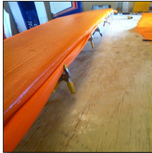
Figure 17 add spring clamps to keep skin from curling
