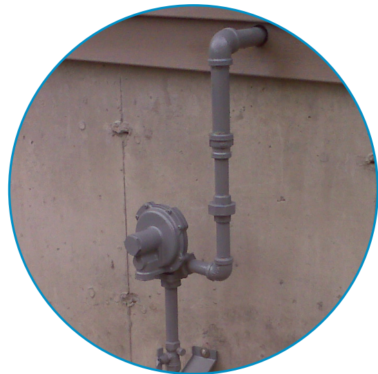
Example of a secondary pressure regulator
