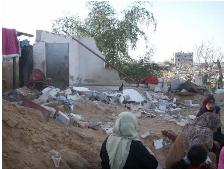
Damage to the Zeitoun neighbourhood (CC BY-SA 2.0)
