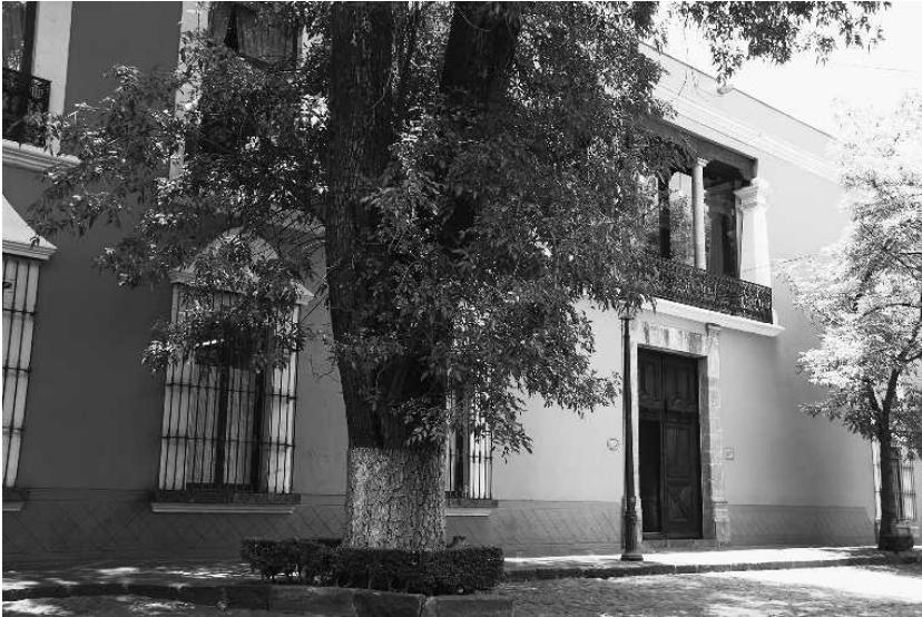
FIGURE 4.3. Former Textile Mill, Coyoacán, Mexico City. A great number of chino slaves worked in this textile mill owned by Melchor Díaz de Posadas during the seventeenth century. Present home of the presidency of the Consejo Nacional para la Cultura y las Artes. Photograph by Alexandra Hart Brown and Daniel Fermin Pfeffer.
